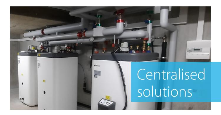
Centralised applications integrate a central source of energy for heating and hot water. Cascade solution is a type of centralised system in which one outdoor unit supplies energy to multiple apartments. Each apartment still includes an indoor unit as control center.
