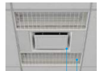
Air discharge outlet from VRV indoor unit Air suction inlet
